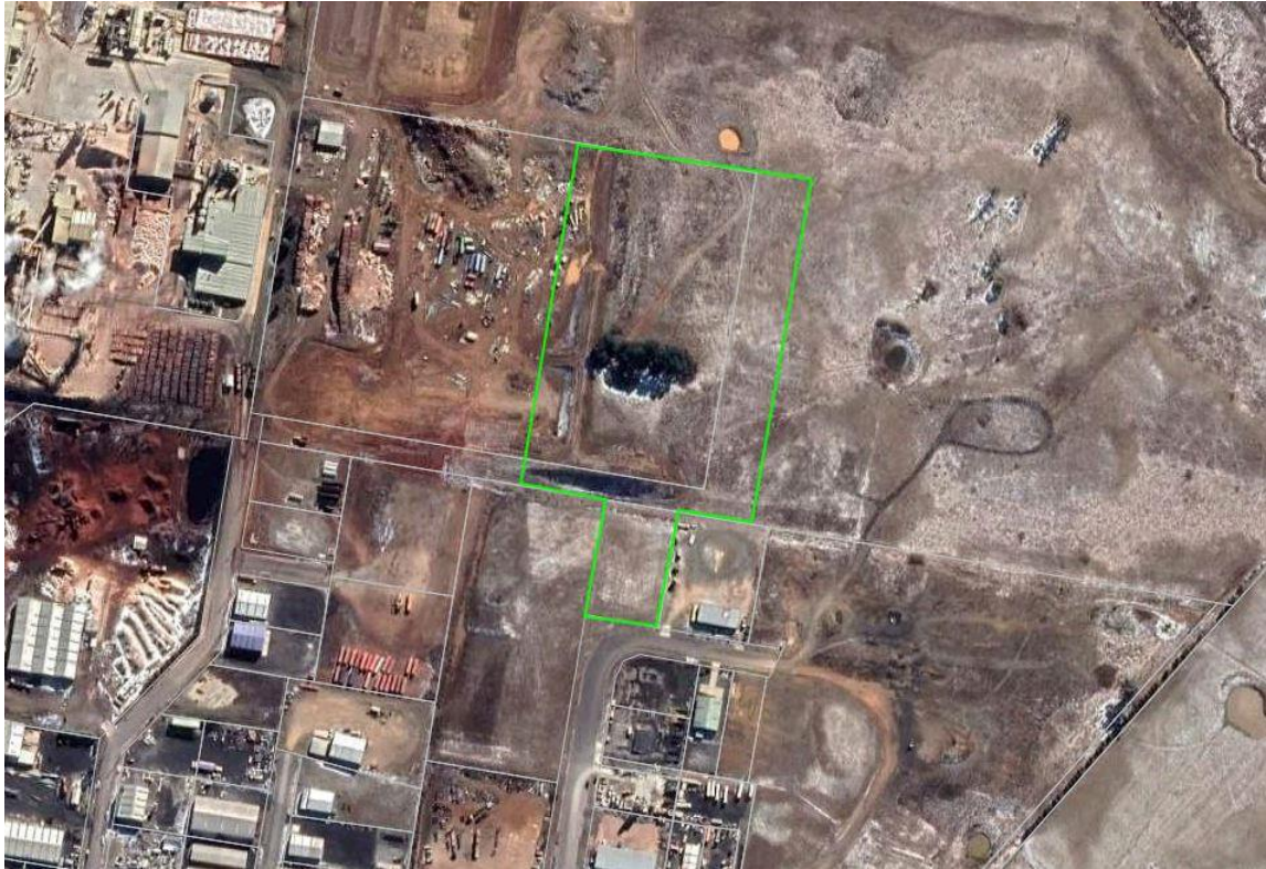
Figure 2 – 2018 aerial image of the approximate development footprint (Green)
